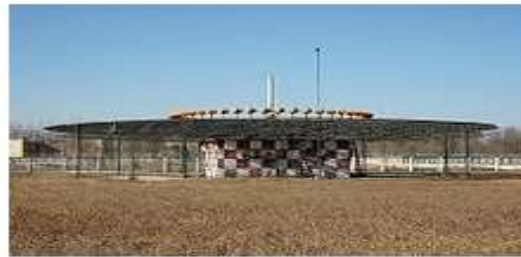
DVOR (Doppler VOR) ground station, co-located with DME
