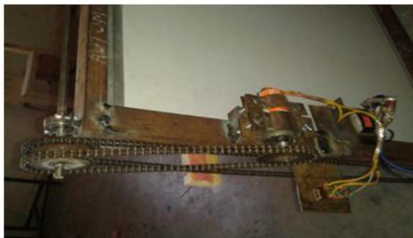
Fig :- Location of motor for power drive
