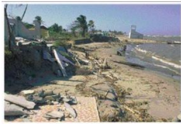
Fig. 1. Aftermath of Hurricane Mitch in 1998 in Northern Honduras [3]
