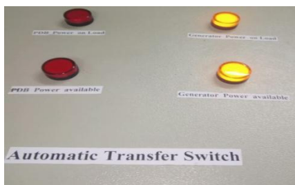
Figure 10: YELLOW LED indicating Generator Power Available / on load
